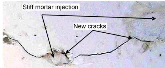
FIG. 1. New cracks of masonry in the area of too stiff strengthening in relation to original strength [6].
