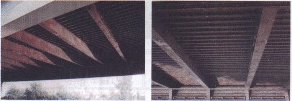
FIG. 4. Details of transverse cross-beams supporting the longitudinally stiffened plate and instrumentation.
