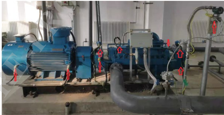
Figure 5. CSDK90-50*10*220kW external pump measurement point layout location
