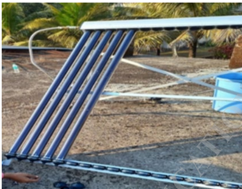
Figure 10. Installation of evacuated tubes at the testing site.
