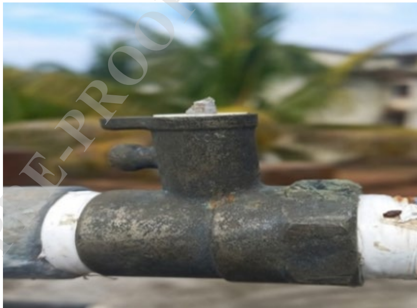
Figure 8. Air relief valve.
