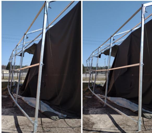
FIG. 7. Visible minor damage to the frame.
