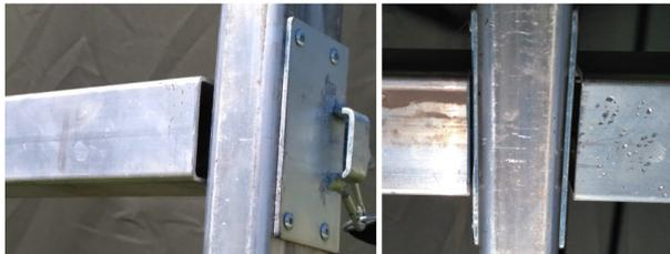
FIG. 3. Method used to connect vertical and horizontal beams mutually.
