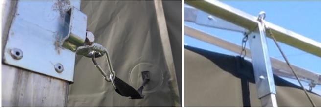
FIG. 4. Connection of the frame to the tent canopy: using webbing (left) and chains (right).
