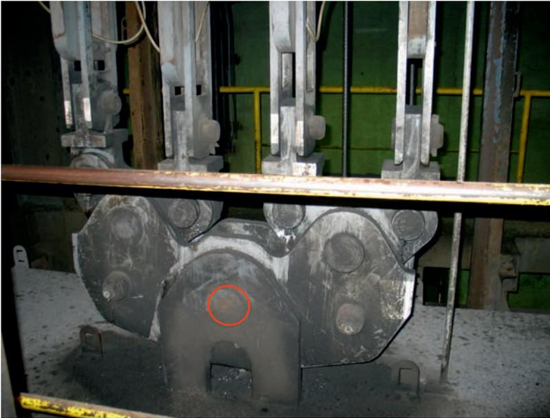
FIG. 5. Attachment of tail ropes for the skip with the support point in the FEM model revealed (red ring).
