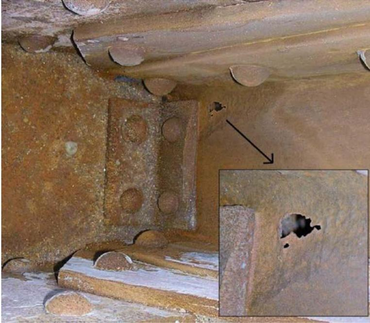
FIG. 1. Corrosion hole in bridge structural element.
