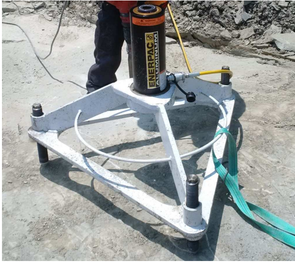
FIG. 19. Pull-out test performed on actual rock.
