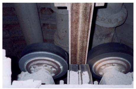
FIG. 13. Roller guide assembly- at the bottom.
